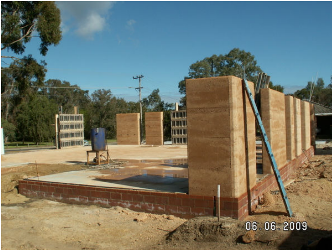
Rammed Earth Walls
