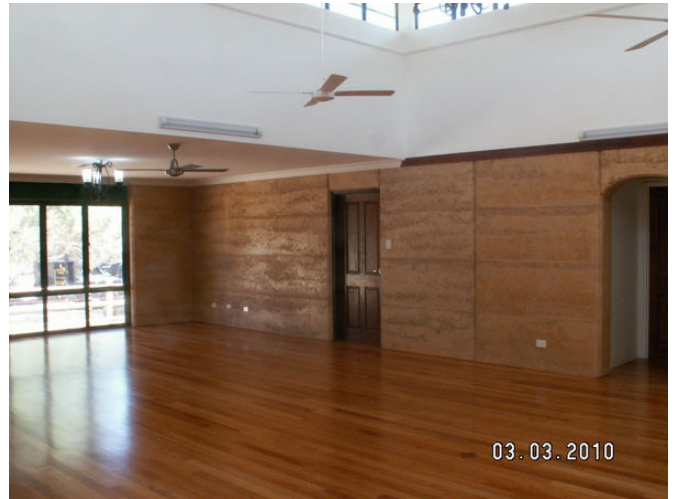
Internal Rammed Earth Walls
